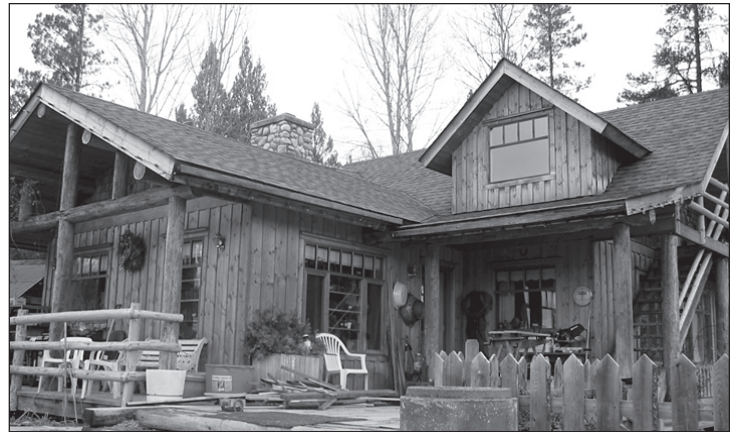
Janet’s house today is beautifully finished, but she still has a pile of old lumber on the porch ready for future projects
